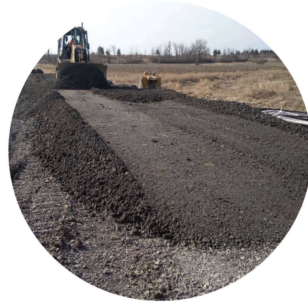
CONSTRUCTION OF ACCESS ROADS, LAYDOWN AND WORKING AREAS
