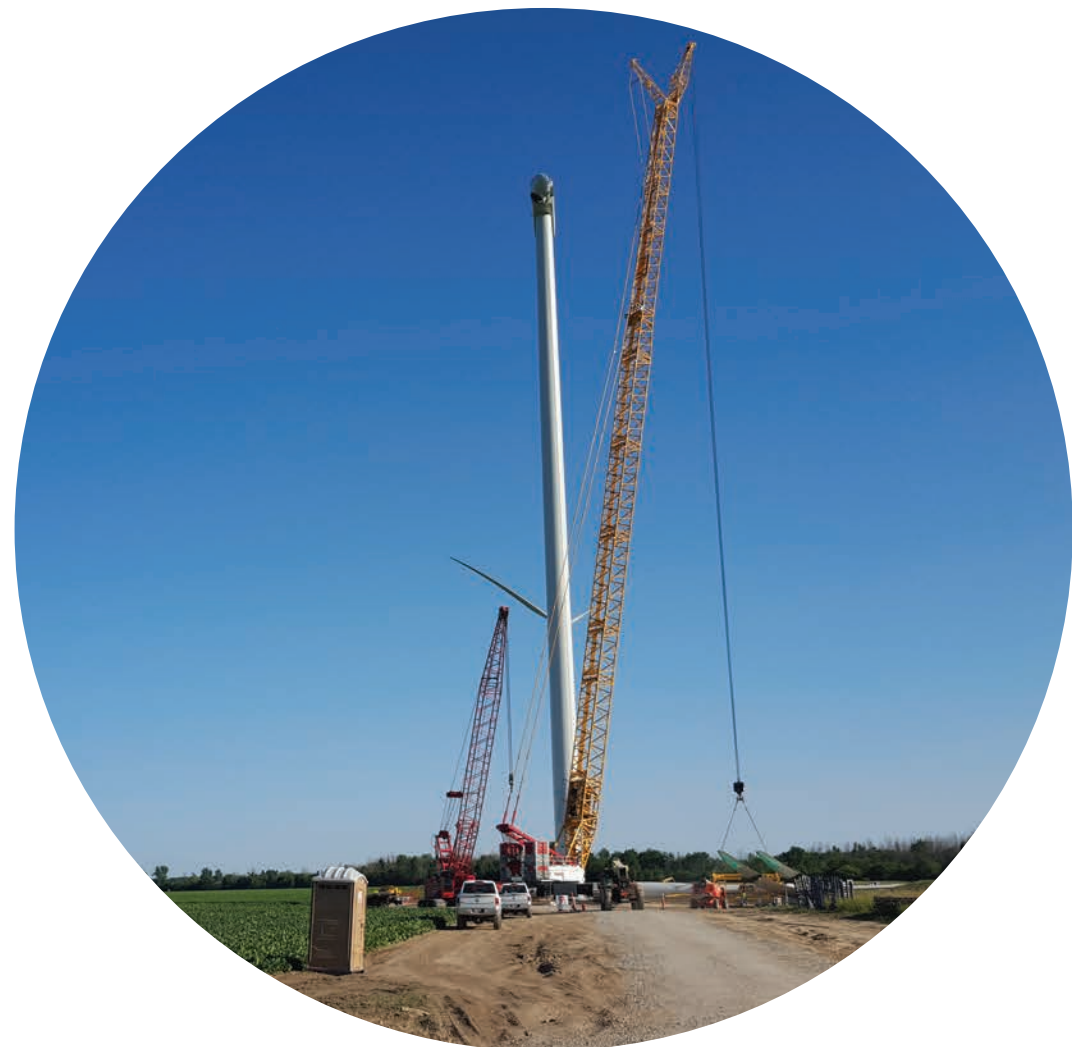
ASSEMBLY AND INSTALLATION OF WIND TURBINES
