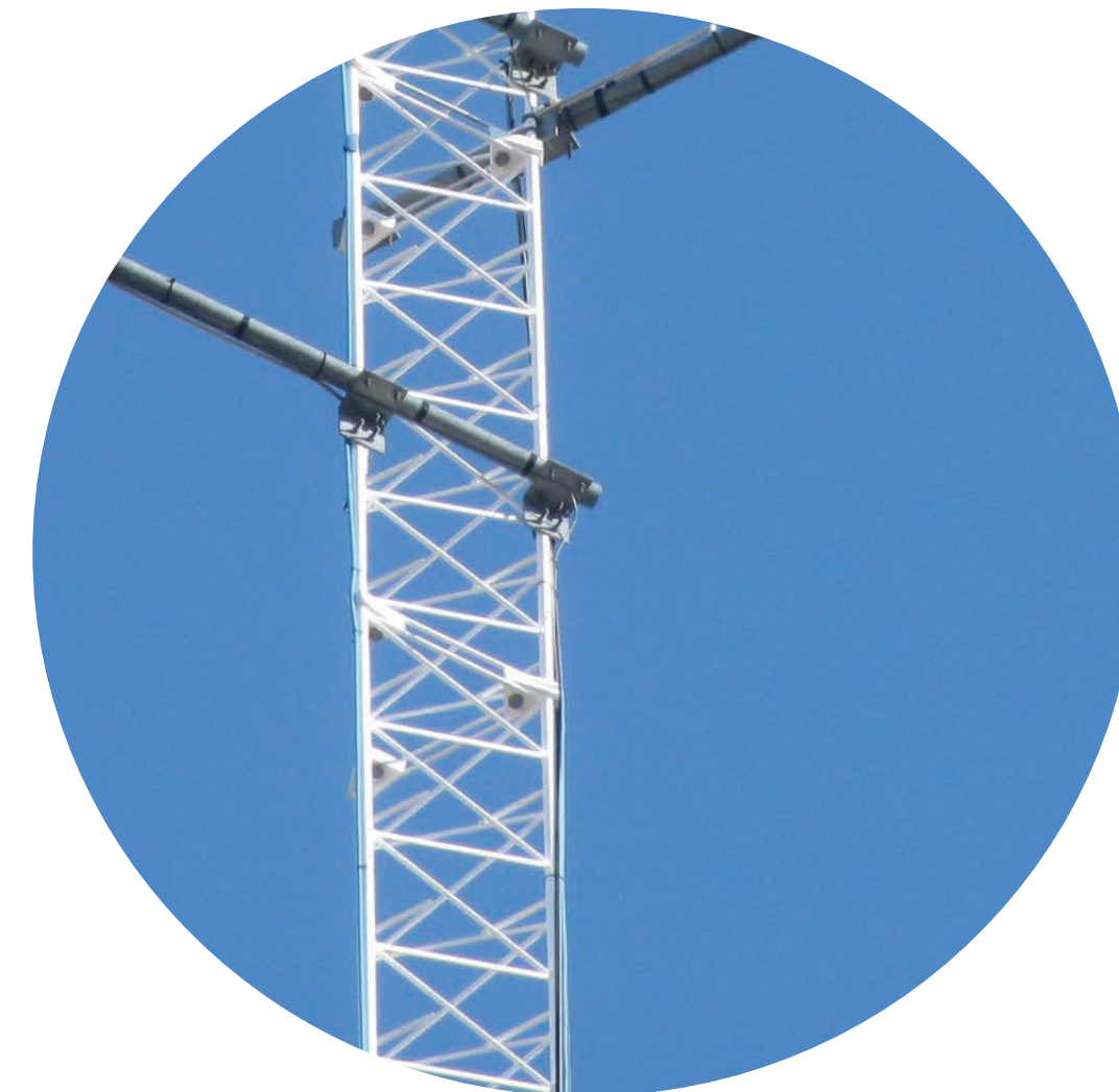
CONSTRUCTION OF COMMUNICATIONS AND METEOROLOGICAL TOWERS
