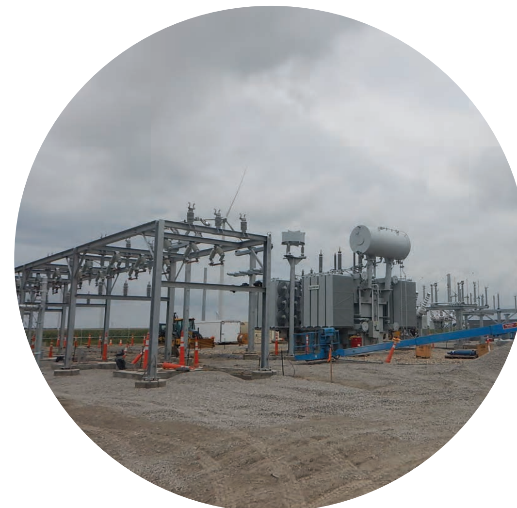
CONSTRUCTION OF ELECTRICAL COLLECTOR SYSTEM, SUBSTATION & INTERCONNECTION POINT
