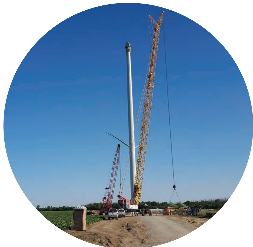
ASSEMBLY AND INSTALLATION OF WIND TURBINES
