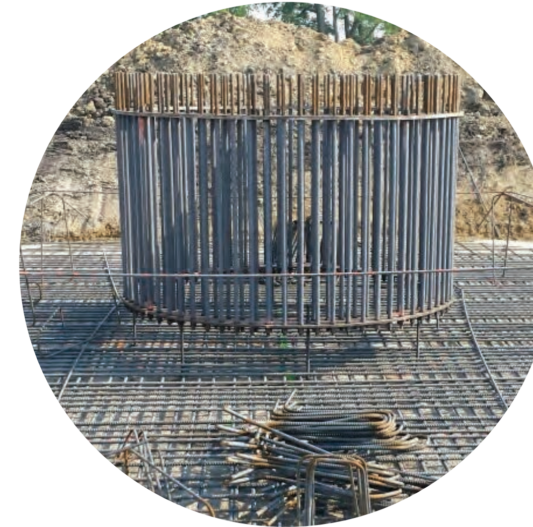
CONSTRUCTION OF WIND TURBINE FOUNDATIONS
