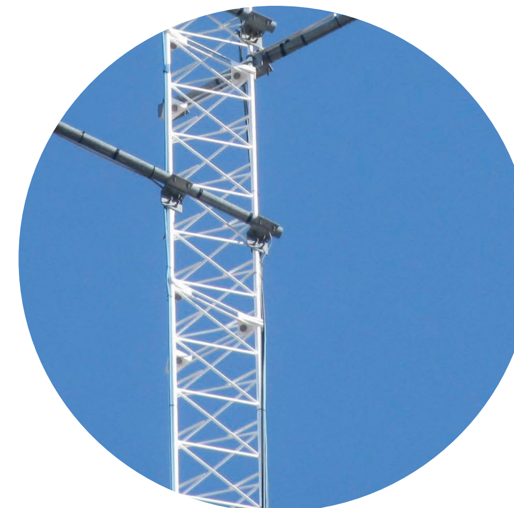
CONSTRUCTION OF COMMUNICATIONS AND METEOROLOGICAL TOWERS
